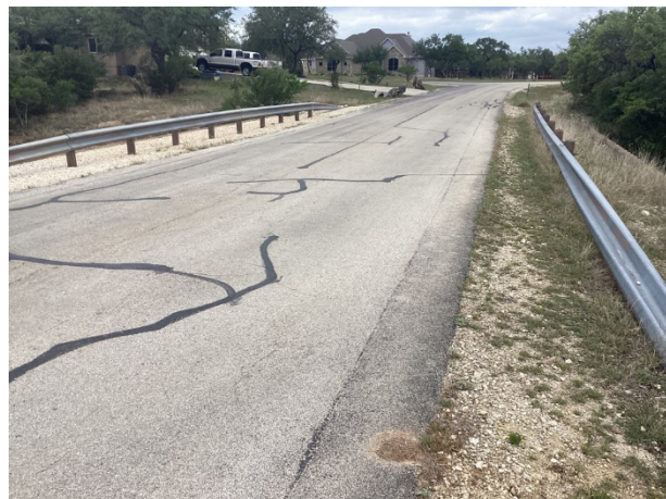
Asphalt pavement street overview
