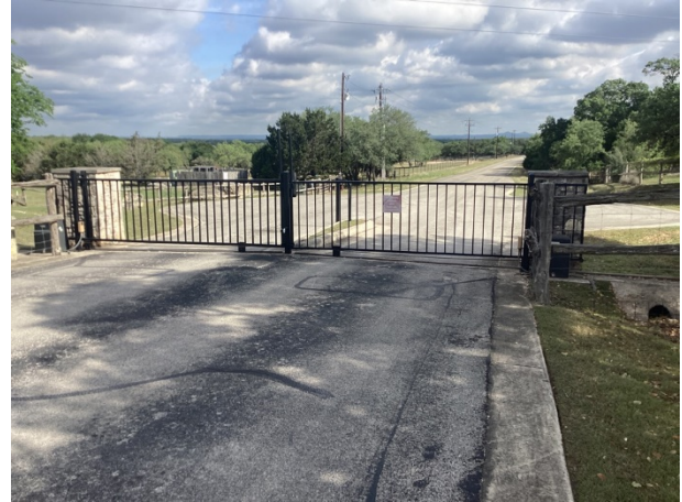
Steel gates at Lantana Canyon
