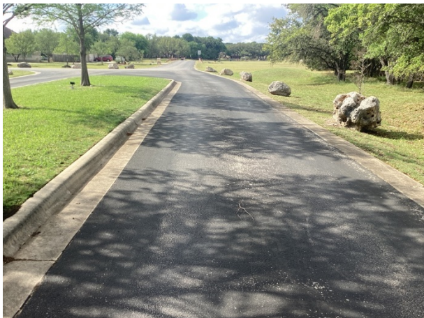
Asphalt pavement street overview
