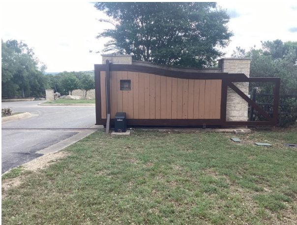
Wood gate with steel frame at Lantana Mesa
