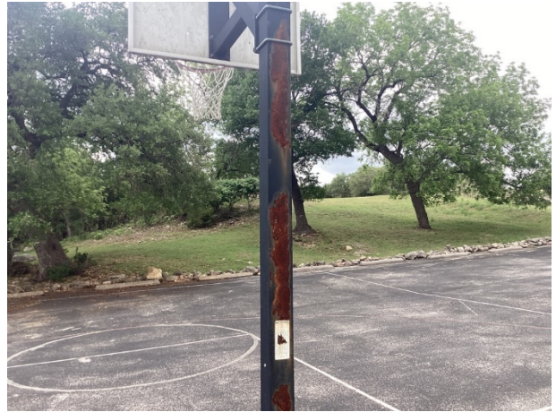
Finish deterioration and rust
