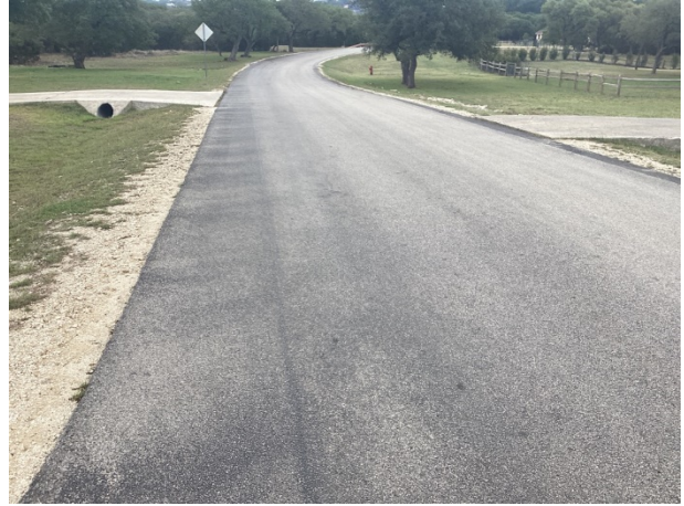
Asphalt pavement street overview
