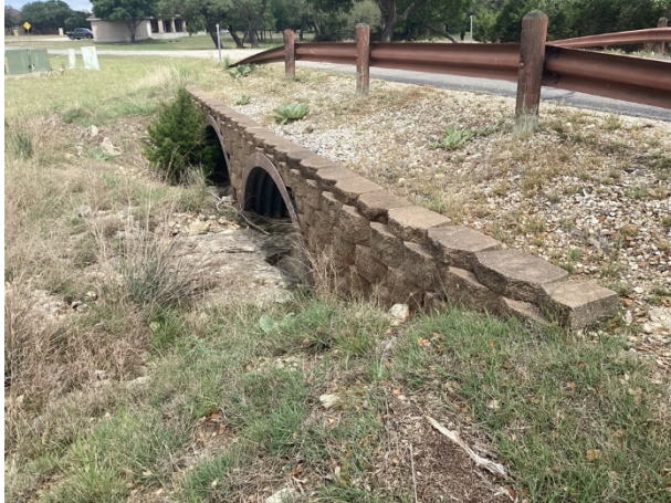
Retaining wall at bridge 3
