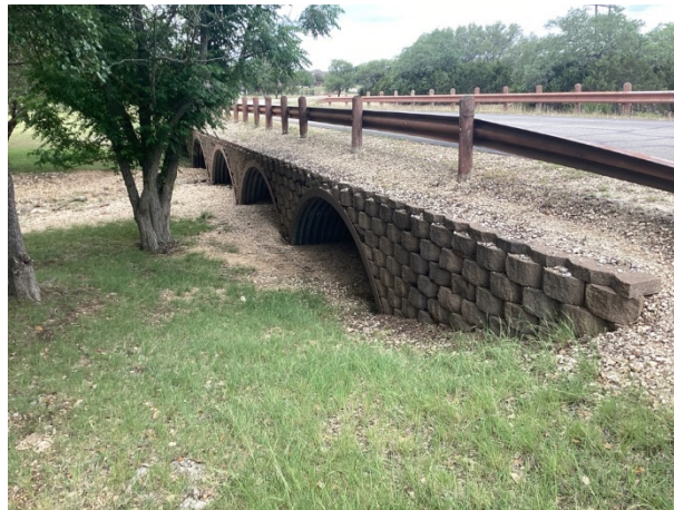
Masonry retaining wall at bridge 2
