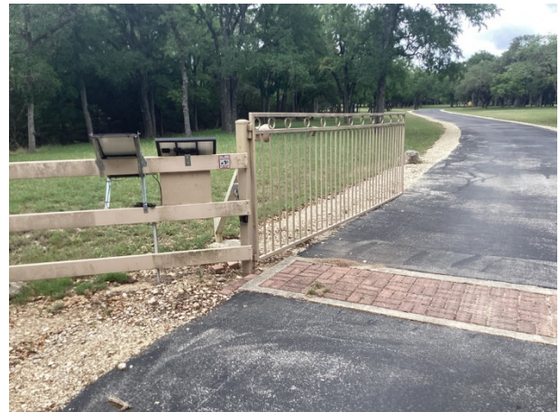
Steel gate at park
