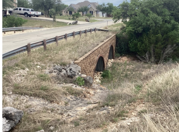
Retaining wall at bridge 5
