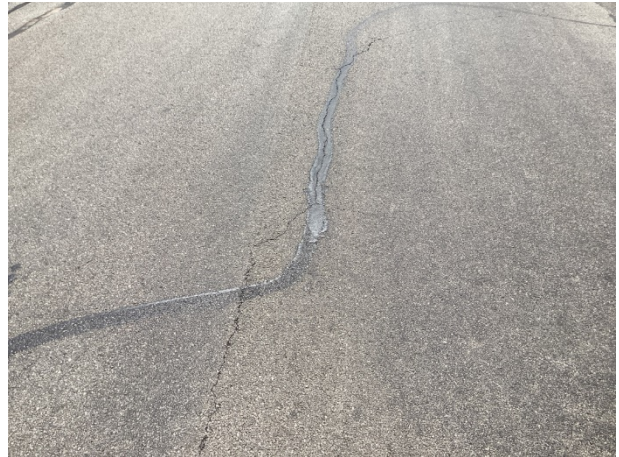
Pavement cracks
