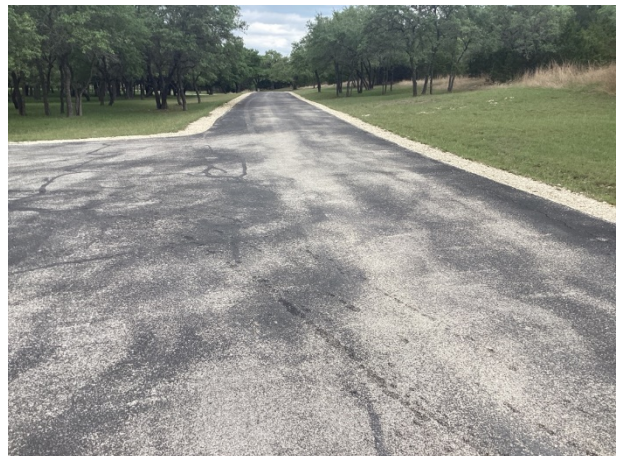
Asphalt pavement park driveway
