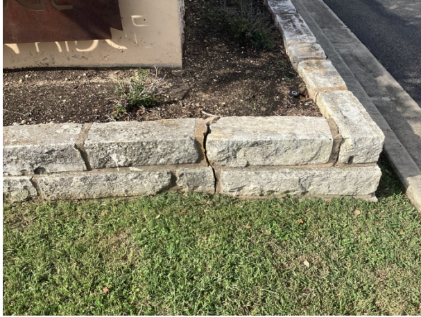
Masonry cracks
