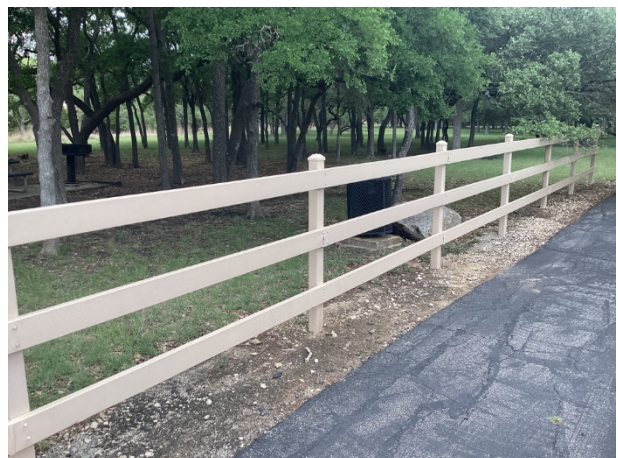
Wood split rail fence
