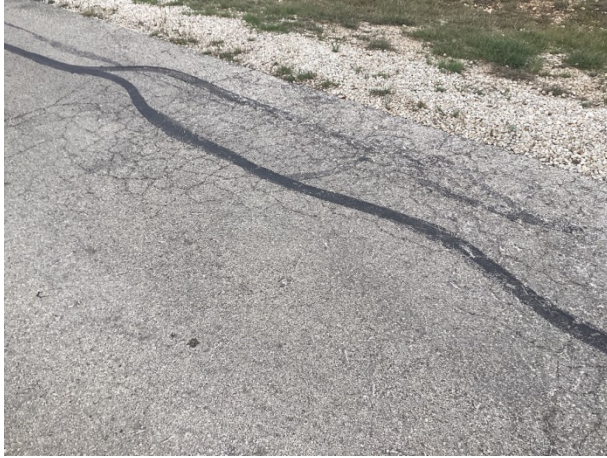
Alligator cracks
